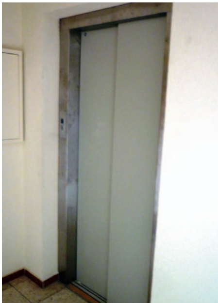
Figure 3: Panelled hinged-door frame with telescopic door
